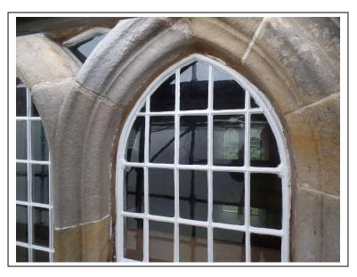
One of the East Gable windows. These were found to be in reasonable condition. There is however a need to properly repair one of the windows where the timber cill had failed and was letting rainwater into the Extension Hall. A temporary repair had already been made, so this work has been deferred until the final Phase of works, as it can be accessed comparatively easily from the Choir Room and Extension Hall roof.
