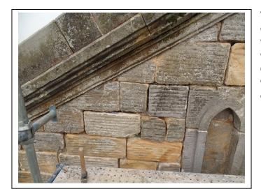
The East Gable wallhead after mortar excavation. It was very apparent that there was a much bigger problem with this wall, as the pointing on the Coursed Rubble stones appeared very much poorer than in other parts of the elevations.
