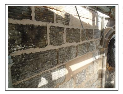
Almost finished. The final lime mortar going into the Coursed Rubble joints. Note how this is left proud of the surface. After a couple of days or so, the mortar has cured enough that flushing off the joints (using a coarse brush) will not cause any damage below the surface.
