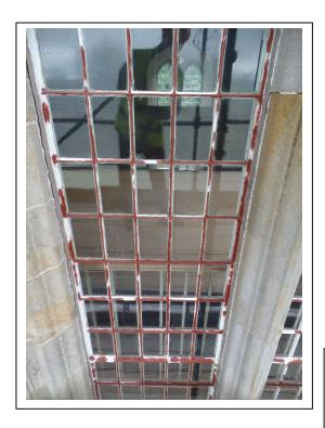
One of the tall windows on the South elevation. These are cast iron. Although cast in at least 2 sections (some were able to be opened), the skill needed to cast these in 1815 must have been immense – it probably couldn't be done today using the facilities available in 1815!
