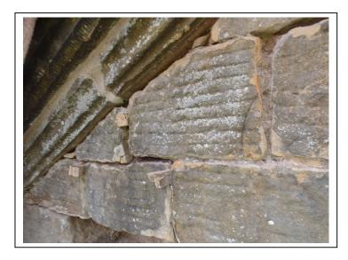
However, it was also apparent that the clay pipes had been bedded in a CEMENT mortar (early examples of this had been in use in Scotland since the mid 1800s), and the removed stones had been replaced using the same material – but very poorly!. This mortar was now crumbling and had no structural integrity whatsoever.
