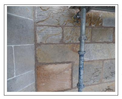
Note matching colouring in the new stone (bottom left) with the old stone. Although the new stone comes from a quarry near Edinburgh, it is thought that this is actually the same stone stratum as in the original quarry in Renfrewshire. This could possibly be confirmed by comparing the chemical and structural compositions from the two stones.
