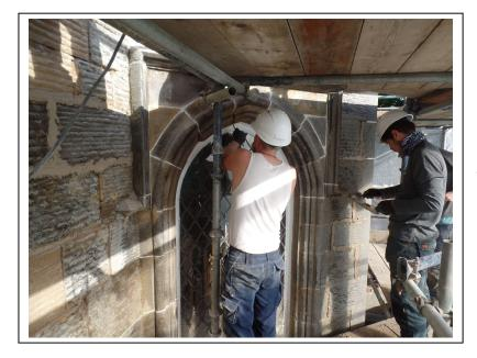
Finishing off the East Gable. This work had been left until the repairs to the wall had been completed. The use of the syringe to inject the white mortar into the Ashlar joints can be seen. Still good weather!
