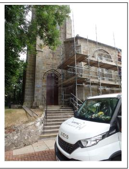
The finished scaffold, now with ant-climb measures and weather protection. Work has started on the top lift.
