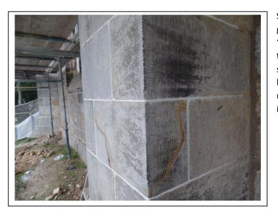
South elevation buttress at ground level. These have been "tooled" lightly using vertical tool marks. The Coursed Rubble stones by contrast have horizontal and deeper tooling marks. Note the coloured veins in the stone.
