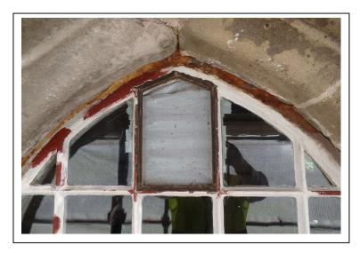
The windows have been scraped to remove loose paint and putty. Red primer has been applied to the bare metal to seal it before new putty is applied. The pointed pane at the top was cracked and has been removed to allow replacement with a new pane. For authenticity, the new glass is from stocks of traditionally made glass.
