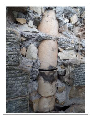
Very shoddy construction of the flue liner! The gaps would allow acidic gases from the coal fire in the Choir Room to penetrate into the wall structure, and then condense to form sulphuric acid, which would in turn hasten the degradation of the mortar packing.
