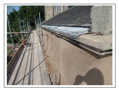
The top lift – coursed rubble pointing complete. The hessian is used to control the rate of drying of the mortar by keeping off sunlight and drying winds. Note the lead at the wallhead – this is a flashing between the bottom of the slates and the cope stones on the wallhead, and also forms a gutter. There is however only one downpipe – rainfall must have been less in 1815!
