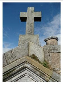
The Cross on the East Gable wall head. It had been thought that the "crack" on the RHS of the base may be loose, but it was found to be only a marking in the stone, and was quite sound. One less job to be done!
