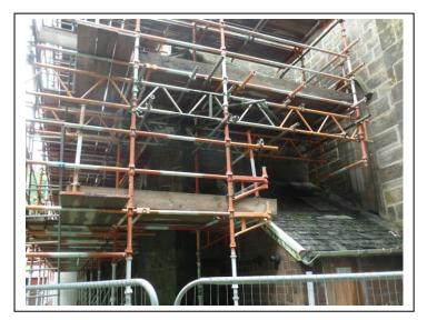
The third lift of the scaffold installed, after much deliberation as to how it could be supported without putting any loading on the Plant Room roof.
