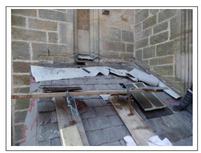
Repairs well under way. The timber "wall head" at the brick wall has been replaced and about a third of the roof sarking boards renewed.
