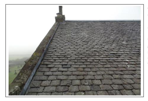
The rest of the roof was checked for loose slates and other potential problems. Most were found to be in good condition but some were crumbling and had to be replaced
