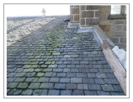
Roof works are about to commence. The main area of concern is at the west end of the roof where rainwater coming from the tower has been directed to run down the slates, increasing their exposure to prolonged dampness and Verdigris growth.
